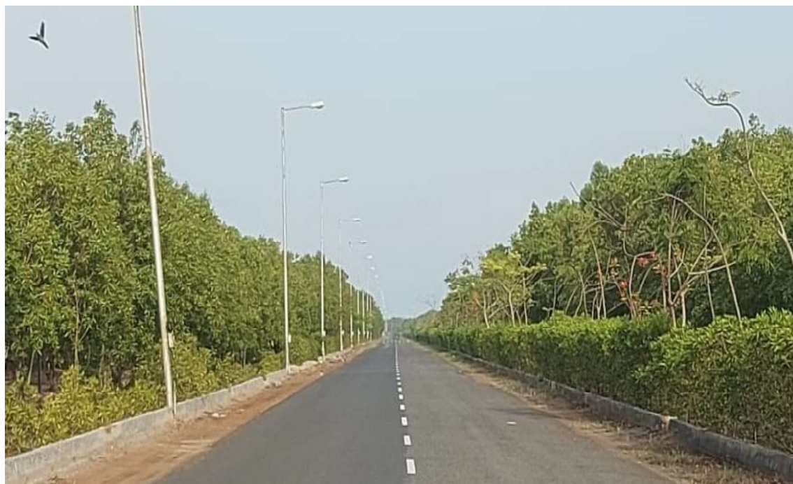
GREEN COVER ALONG PIPE RACK & INTERNAL ROADS
